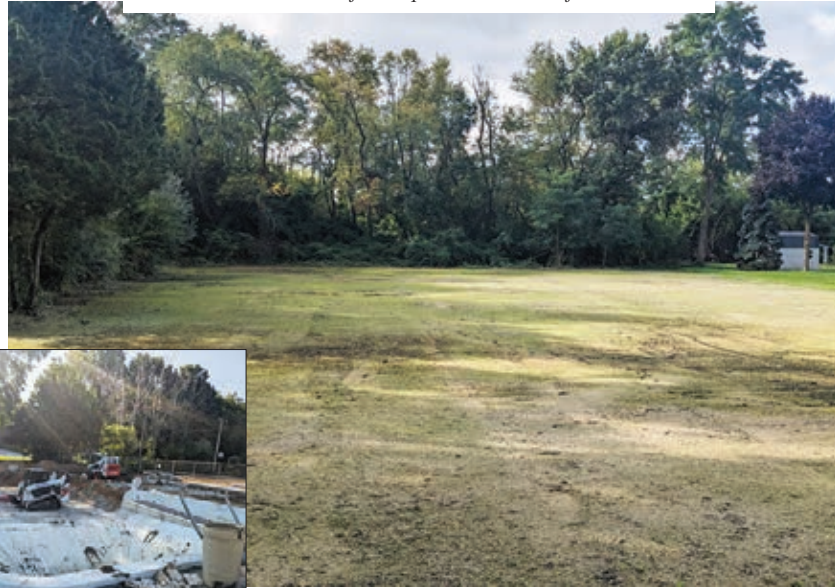
1169 Robinhood Drive former pool and courts - after renovation.
