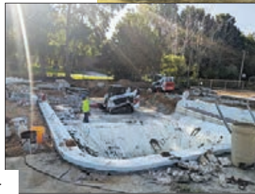
Sherwood Oaks former pool on Robinhood Drive - during renovation.
