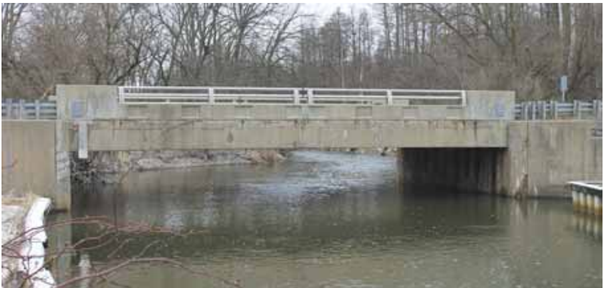
Facilities and Road Maintenance has been working closely with Cook County Department of Transportation and Highways, and has begun the process of planning for the required Rohrssen Road bridge over Poplar Creek replacement. The project is expected to take five years to complete, with construction beginning in 2029.
